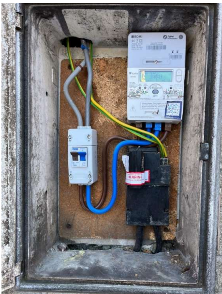
Figure 2.3a Looped supply with external meter box
