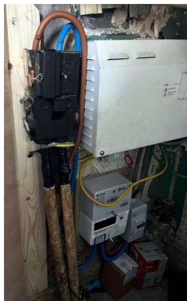
Figure 2.3b Looped supply with internal DNO cut out and meter
